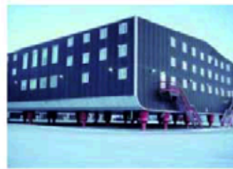
BP operations center, Prudhoe Bay, Alaska, built on pilings to resist damage from thawing permafrost.
