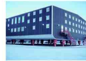
BP operations center, Prudhoe Bay, Alaska, built on pilings to resist damage from thawing permafrost.
